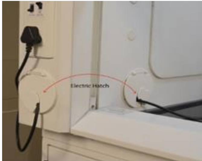
FIG: 16 TYPICAL ELECTRICAL HATCH DETAILS
